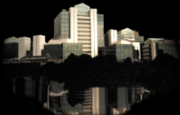
Offices and apartments adjoining the river Thames, East London Use of various bearings to accommodate structural movement
