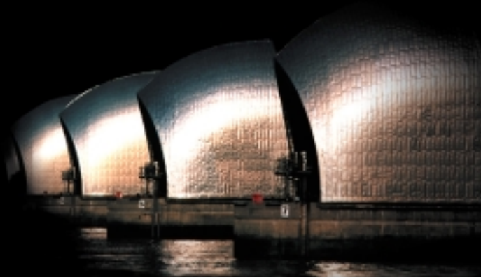
The Thames Flood Barrier, London Use of special SKS sliding bearings
